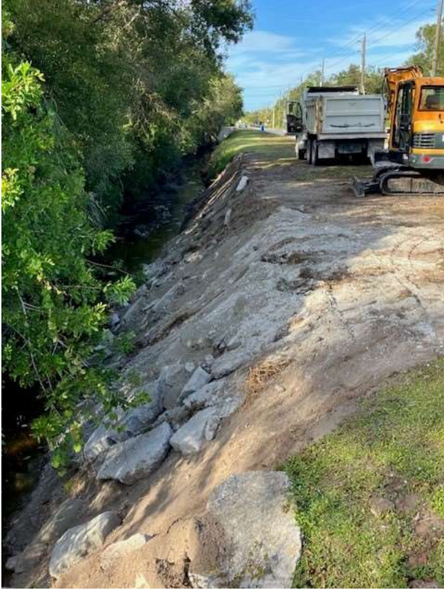
After Completed Repairs
