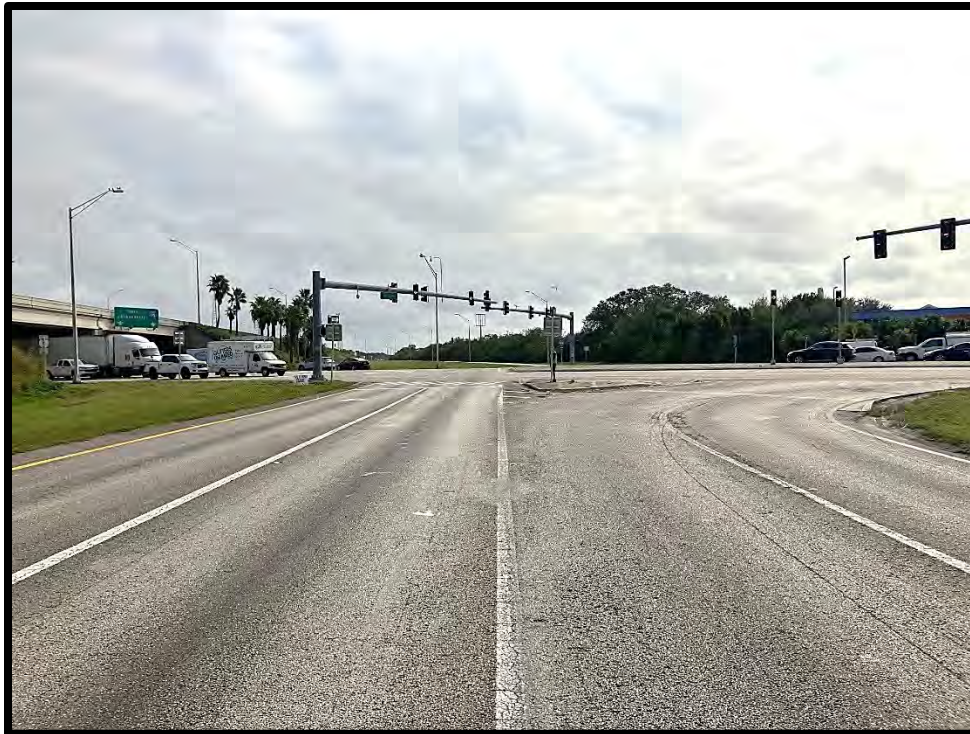
Looking South Towards Intersection
