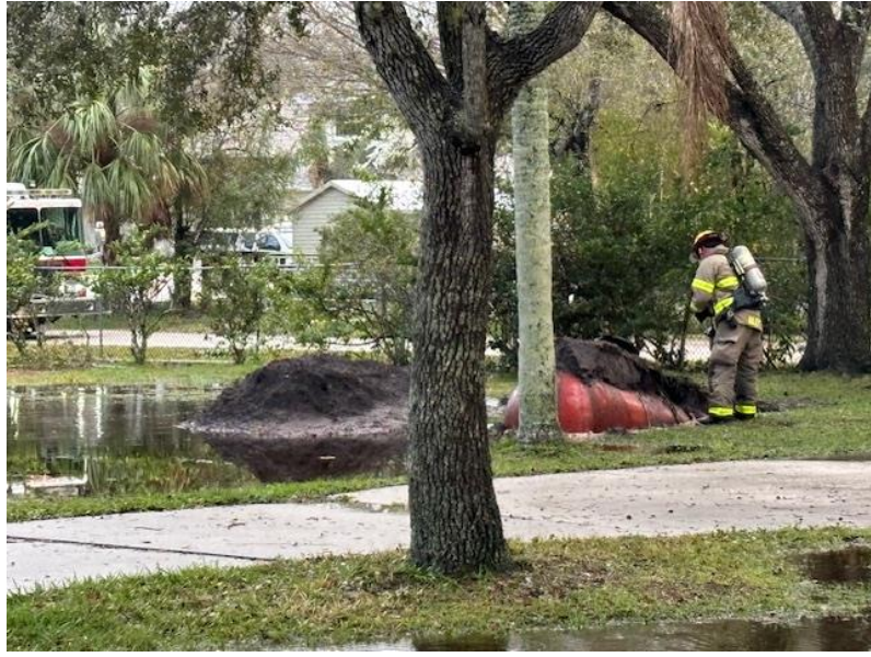
Response to a buried propane tank that broke the surface after significant rain. E99 crew worked to assess for any leaking from the tank. Crews' shutdown the valves from the tank leading into the house. Scene turned over to the gas company.
