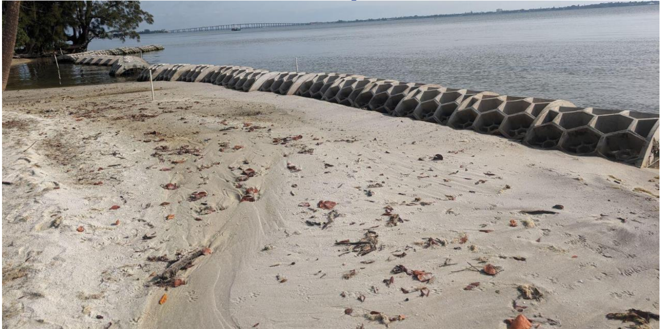
Figure 6. Within four weeks of deployment, the MRC Reef Arch living shoreline has built up 15 feet of horizontal sediment and nearly 4 inches of vertical sediment. Fish, birds, rays, and other wildlife have been observed using the arches as habitat.
