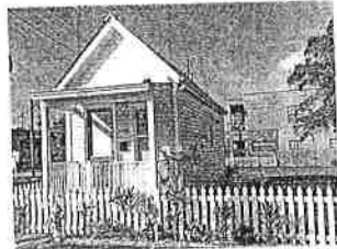
David Bailey built this tiny house, shown Jan 23 in Ybor City, and plans to break ground on a second soon. It has 365 square feet on the ground floor and a small loft for a home office above. Rental demand through Airbnb has been strong, he says. RICHARD DANIELSON, TAMPA BAY TIMES/AP
