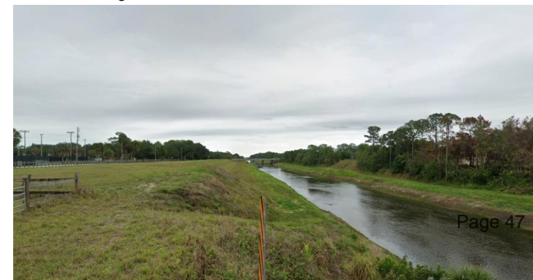
C-1 Canal in Palm Bay Source: Google Earth
