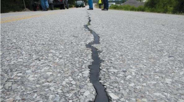
CRACK SEALING
