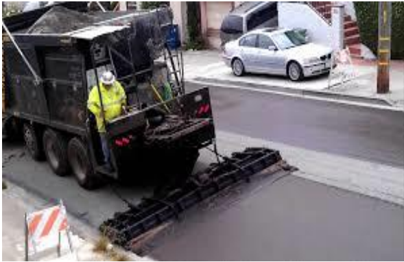
SLURRY SEALING
